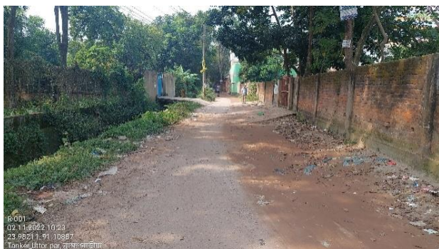
Road-001, Brahmanbaria Paurashava
