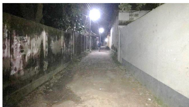
Road-013, Brahmanbaria paurashava
