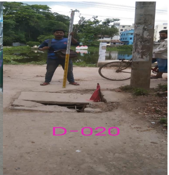
Photo , Haziganj- Drain -20
