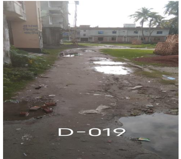
Photo , Haziganj- Drain -19
