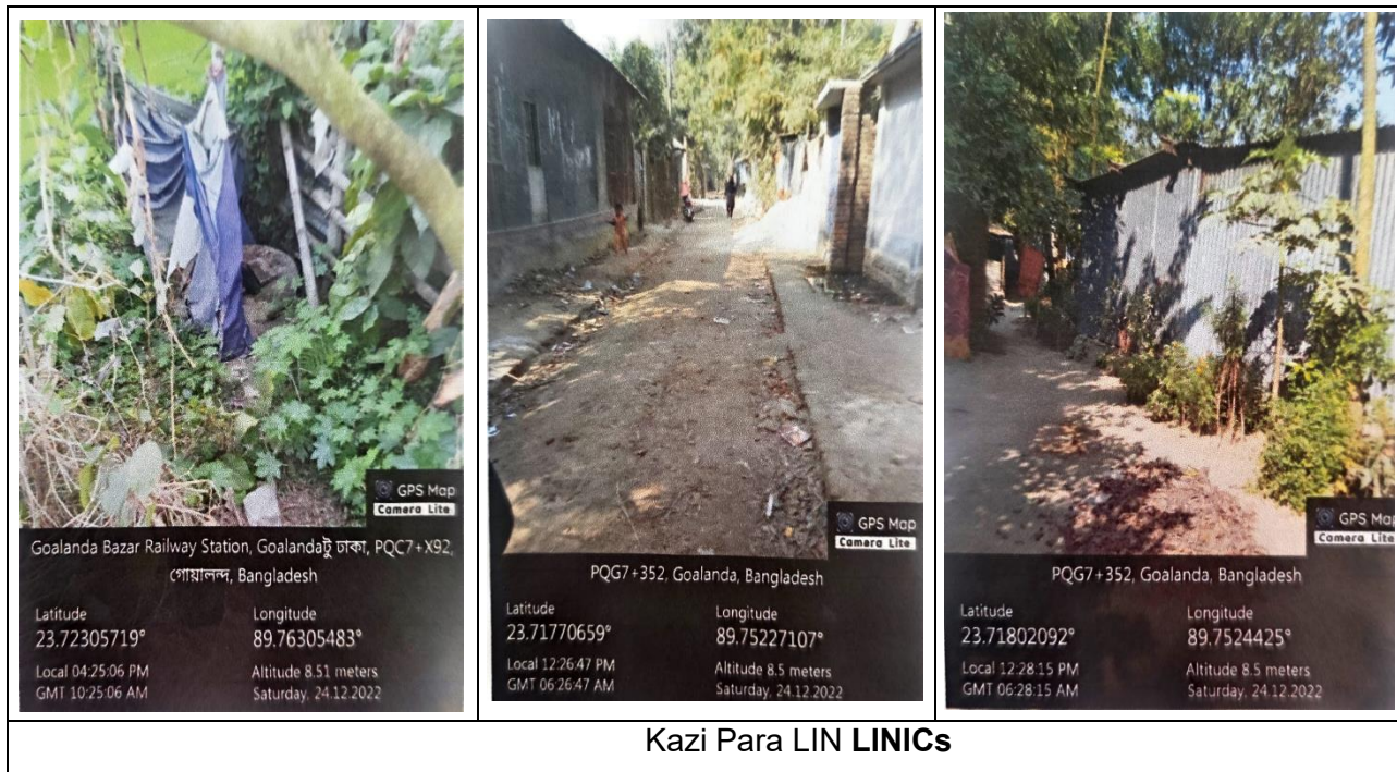
Figure IV.1: Existing Situation at Kazi Para LIN
