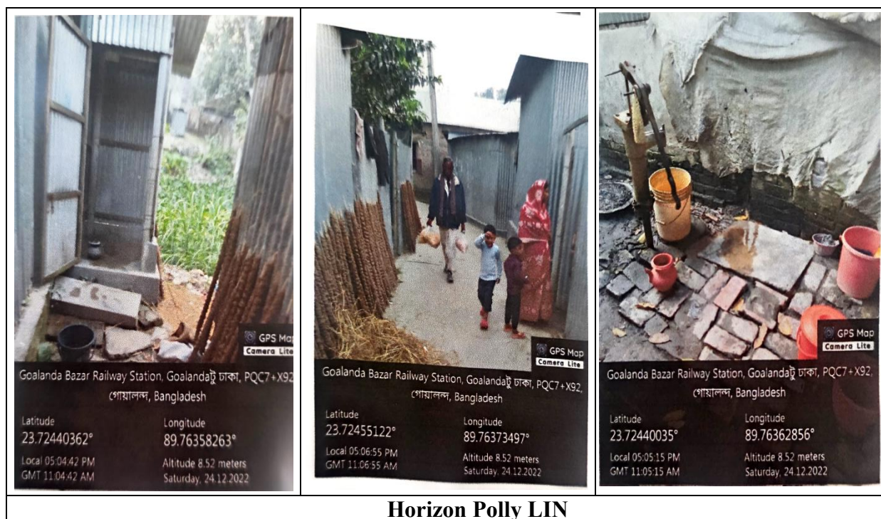
Figure IV.2: Existing Situation at Horizon Polly LIN
