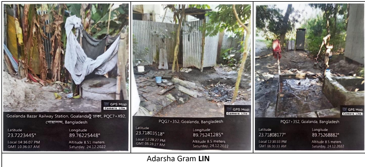
Figure IV.5: Existing Situation at Adarsha Gram LIN
