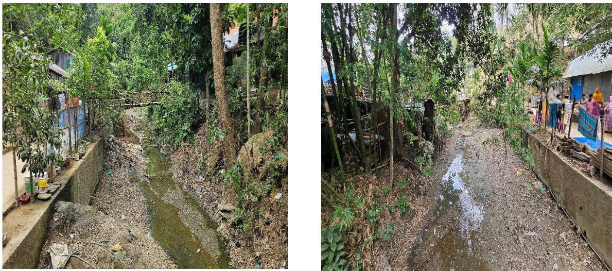
Figure 3-3: Existing Condition of Proposed Khal
