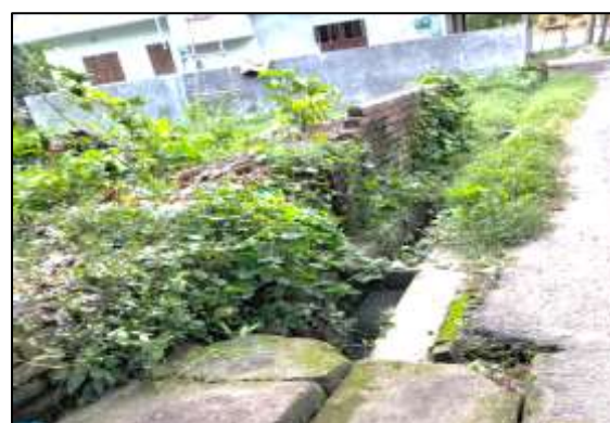
BHER -D-16: Construction of RCC Drain beside Hirimdia Road to Chandona River (Ch.0.00m to 794m) at Ward No. - 03, Bheramara Pourashava, Kushtia.
