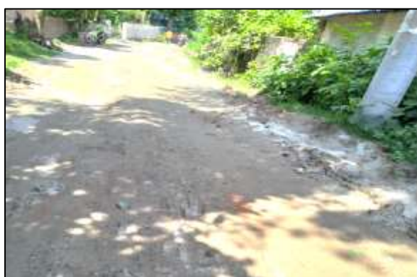
BHER R-16: Improvement of road by Dense Bituminous Carpeting Road a. from SDO house to Amla Road (Hirimdia road) at Ward no. - 8, Bheramara Pourashava, Kushtia.
