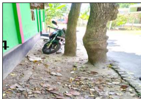
BHER -D-04 Construction of RCC Drain from H/O Ekram to Proposed Drain D - 01, Part - B: Construction of RCC Drain from H/O Ekram to existing drain near Nurjahan Road, at Ward no. - 02, Bheramara Pourashava, Kushtia.
