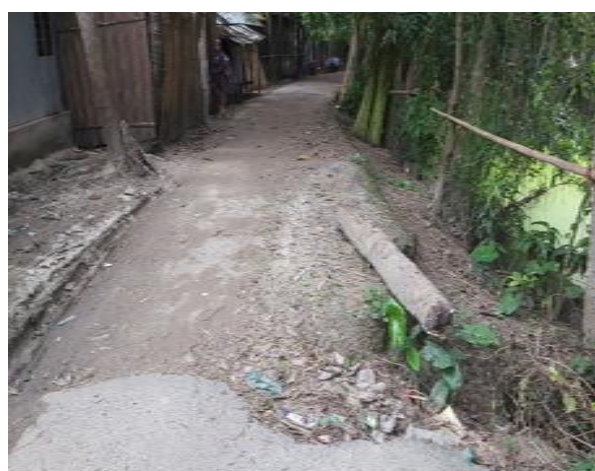
BOAL-R-13: Improvement of Road by DBC from Chatul R&H Road near Fire Service to Loknath end of Paurashava boundary via Mannan Councilor house (Ch. 0.00-1550.00m) & RCC (Ch. 1550.00-1827.00m), Protection Work 58.00m. at Ward no.-08 & 09 Under Boalmari Paurashava, Faridpur. (Total Length=1827.00m).
