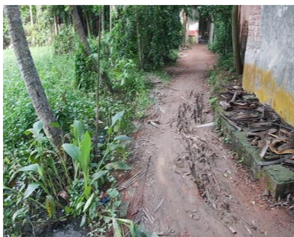
BOAL-R-12: Improvement of Road by Uni-Block Paver Starting from RHD Road to Kriti Ronjon House via New Model School Ch. 0.00-100.00m, Protection Work 20.00m at Ward no.-05 Under Boalmari Paurashava, Faridpur. (Total Length = 100.00m).
