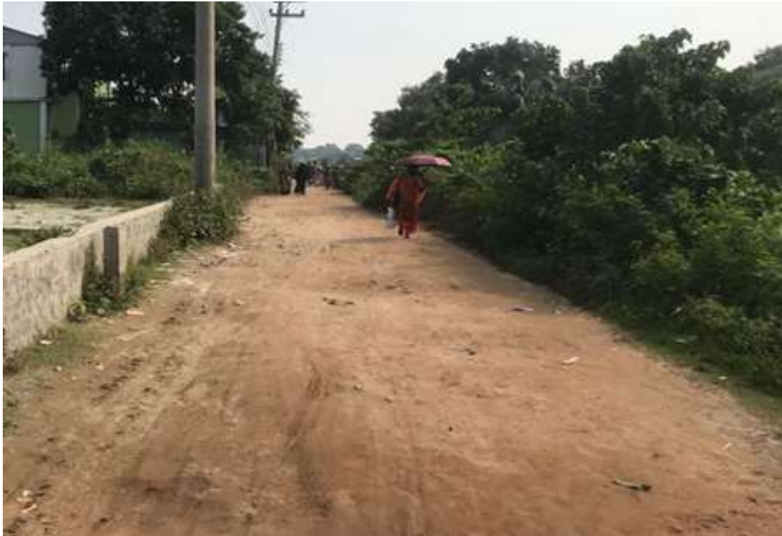
BP-R-06: Improvement of road by Dense Bituminous Carpeting (DBC), starting from Aminpur to Nayanpur via Chandalkhil at Ward 7, Brahmanbaria Paurashava, Brahmanbaria
