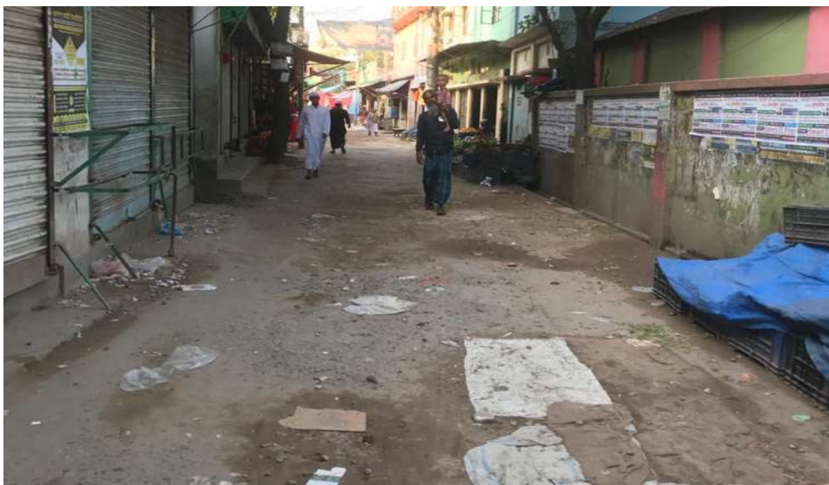
BP-R-08: Improvement of road by Dense Bituminous Carpeting (DBC), starting from Mourail Dakbangalow road to Puniout main road. at Ward no - 9, Brahmanbaria Paurashava.
