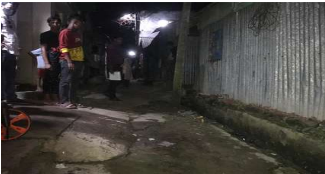
BP-D-09: Construction of RCC Drain at Kazipara, (a) starting from Dhobabari mour to Town Khal at Ward 8, Brahmanbaria Paurashava, Brahmanbaria.
