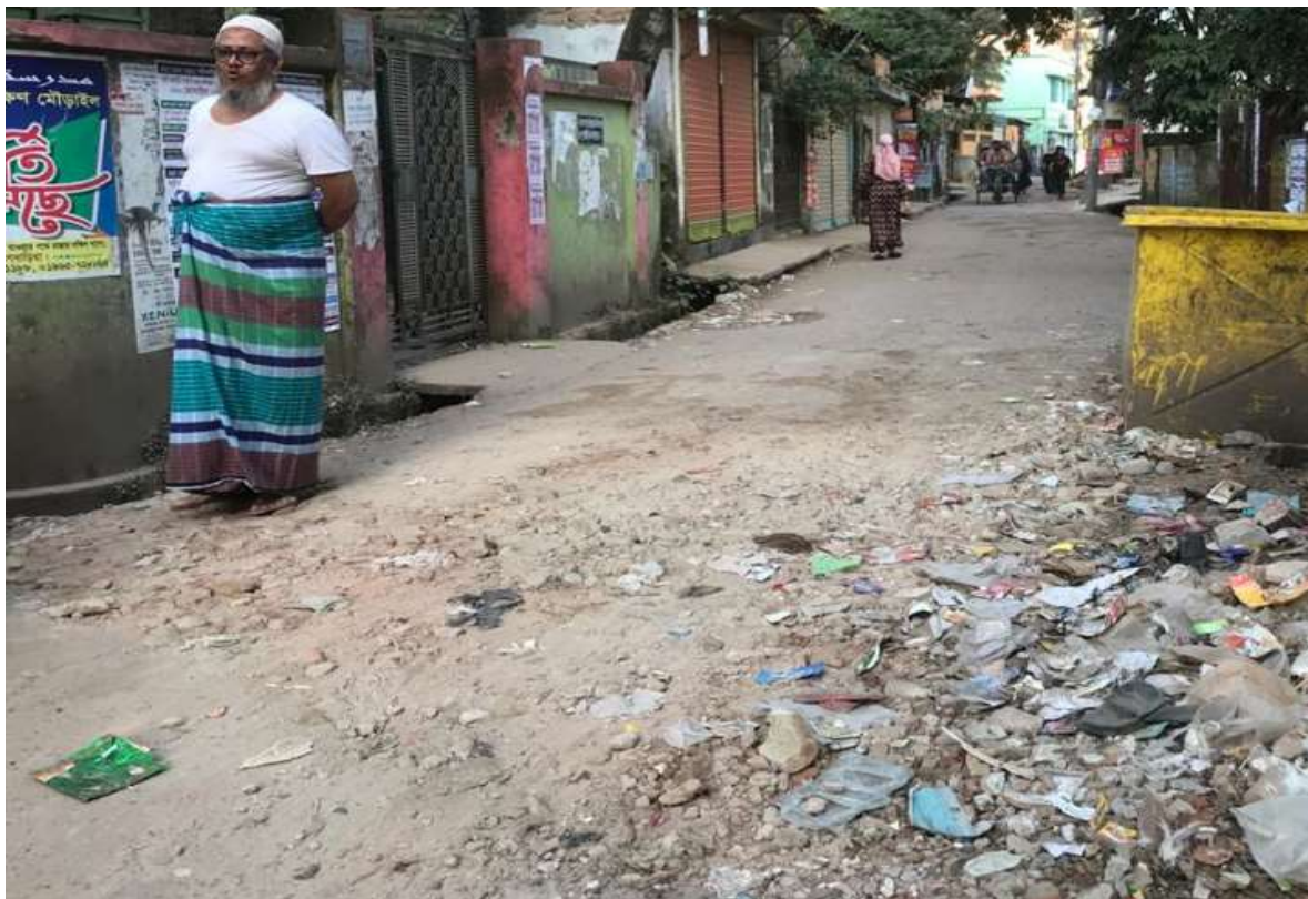
BP-D-10: Construction of RCC drain, (Part- A) starting from right side of Graveyard at Murail Dakbangalow road to existing drain near Land Office at Ward no - 09, Brahmanbaria Paurashava, Brahmanbaria
