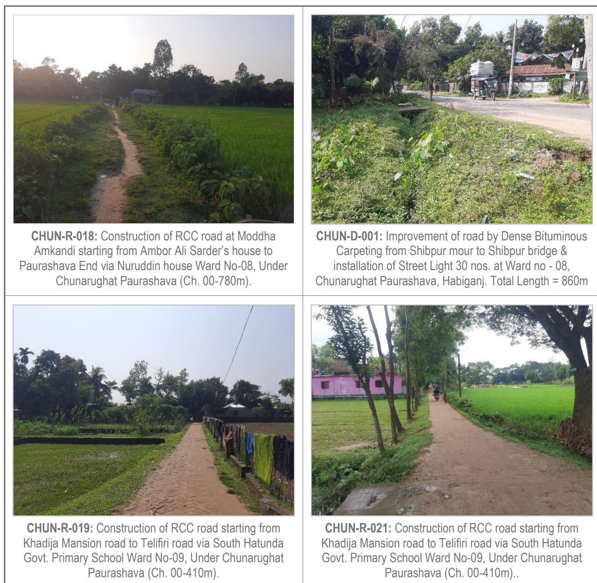
Figure 4: Existing Conditions of Pourashava Roads & Drains
