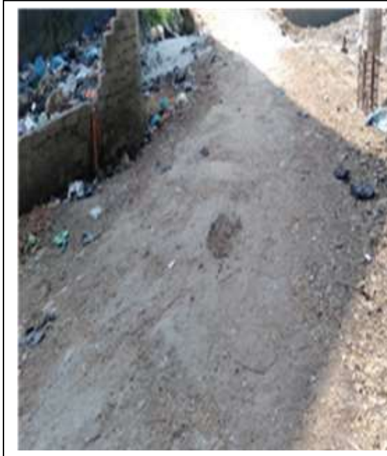
R-31, 32: Improvement & Widening of Shaheed Milon Road Part 1: starting from Haji Ruhul Amin Road to Feni Chowmuhoni road by DBC (Ch.0.00-383.00m) Part 2: Eidgha Road starting from Feni Chowmuhoni
