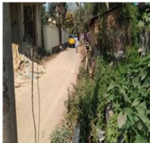
DR-22: Construction of RCC drain lecside Eid gha road starting from Feni chowmuhan road to canal lecside Hazi Ruhul Amin Road (Ch.0.00-436.00m) at
