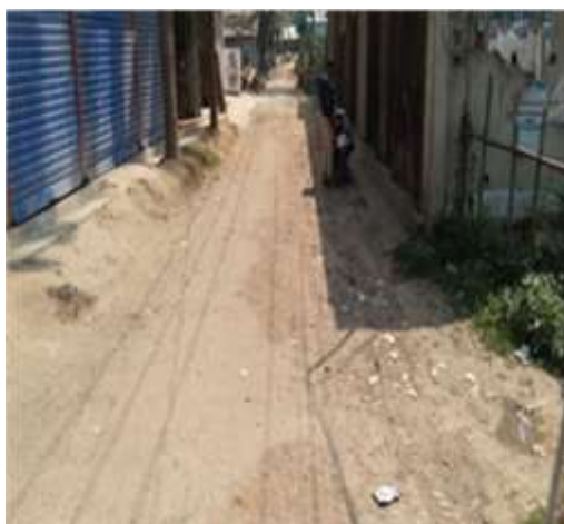
DR- 34: Construction of RCC Drain lecside Bashurhat-Alipur road starting from Taramia Bari to Box culvert near canal (Ch.742.00-10.00) at ward no.03
