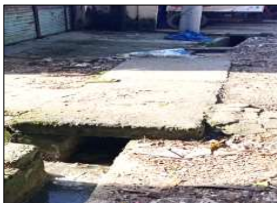
FP- D-078: Construction of RCC Drain beside Kalir Bazar Road to existing Culvert (Ch. 0.00m to 335m) at Ward no. - 07 & 08, Faridganj Pourashava, Chandpur.
