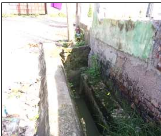
FP- D-081: Construction of RCC Drain from Karim Box Patwary Road to Dakatia River via Police Station and AC Land Office Gate (Ch. 0.00m to 510m) at Ward no. - 08, Faridganj Pourashava, Chandpur.
