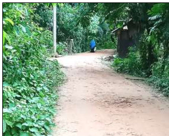
FP- R-264 Improvement of road by RCC from Faridganj - Chandpur Road toward East Safua Kha Bari road through Kachiari Bhuiyan Bari Road at Ward no. - 07 & 08, Faridganj Pourashava, Chandpur.
