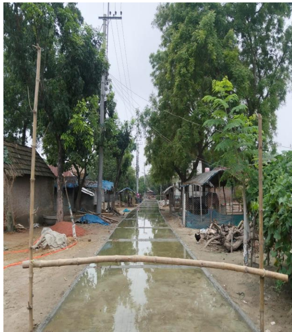
Curing of RCC road in Rohanpur pourashava site
