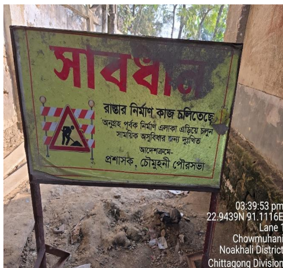
Safety sign in choumohani pourashava site
