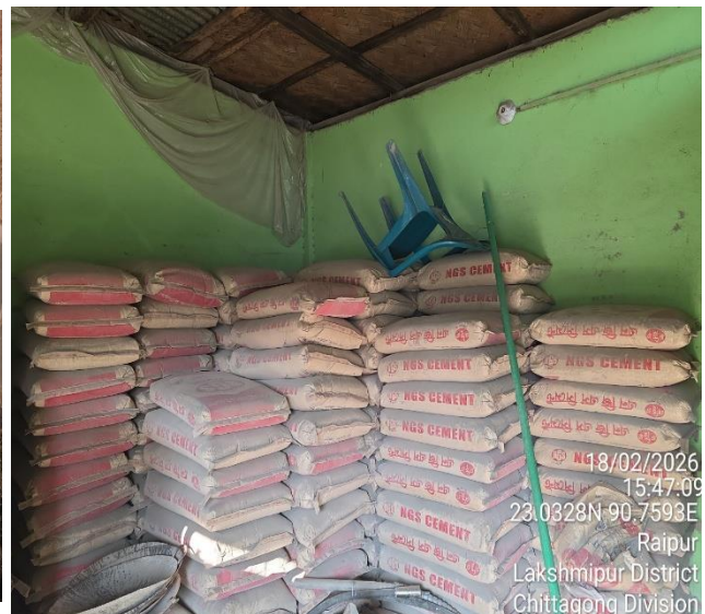
Material store house in Haziganj Pouashava site
