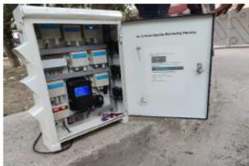
Figure 6: Noise Quality at R-14 of construction site.
