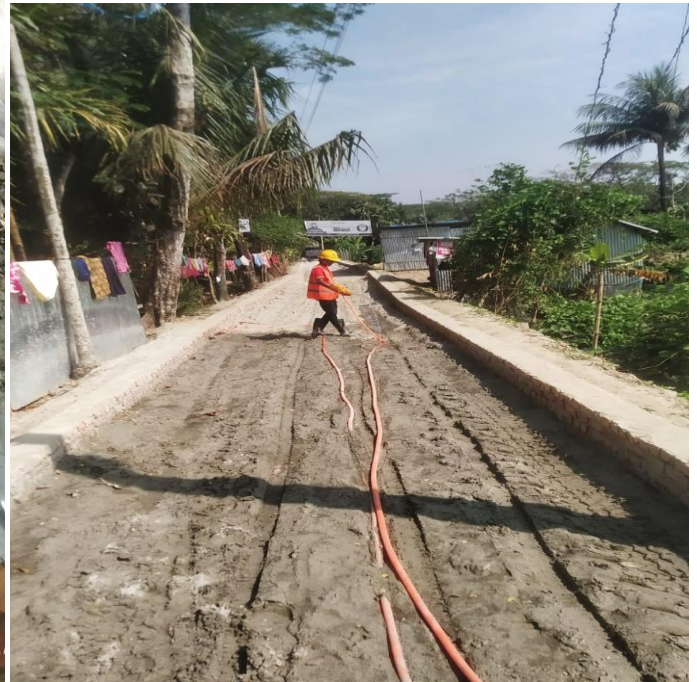
Water spray in Ramgati pourashava site
