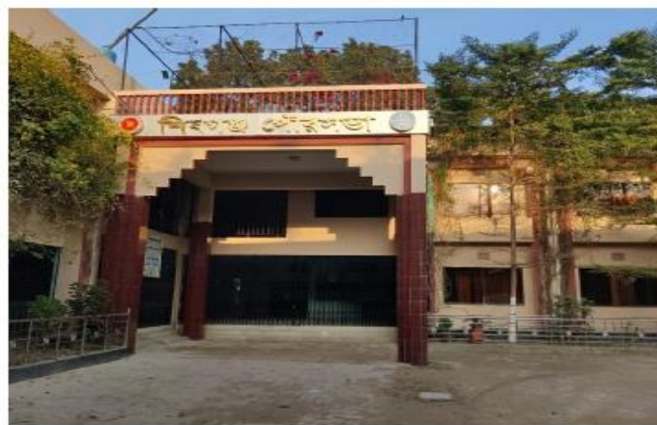
Figure 2 Shibganj Pourashova Building
